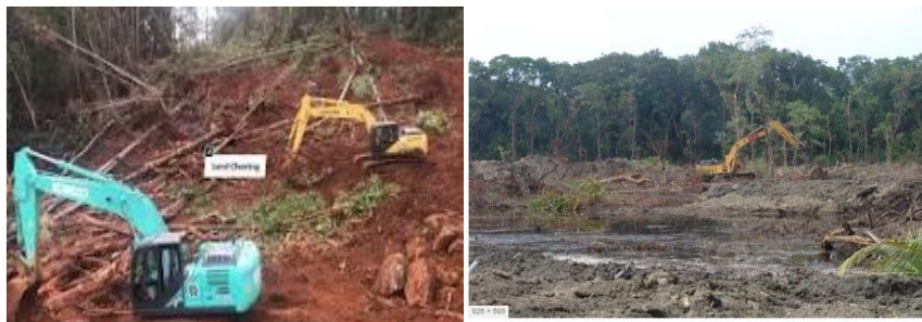
Figure 1. Land Clearing Activities in Block D
